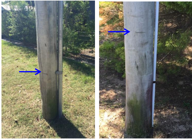
▲ Flood marks in Broulee from 1974
